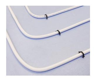
The buildings with irregularly shaped rooms, where the castellated panels with surface bosses limit the correct laying of the piping, enhance the pipe fixing system with clips and Tacker.
